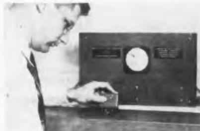
Fig. 5: Checking plating of L-band waveguide
