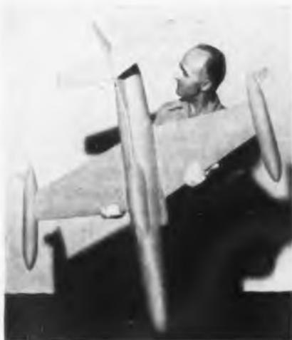
Fig. 3: Jet model has copper metallized skin
