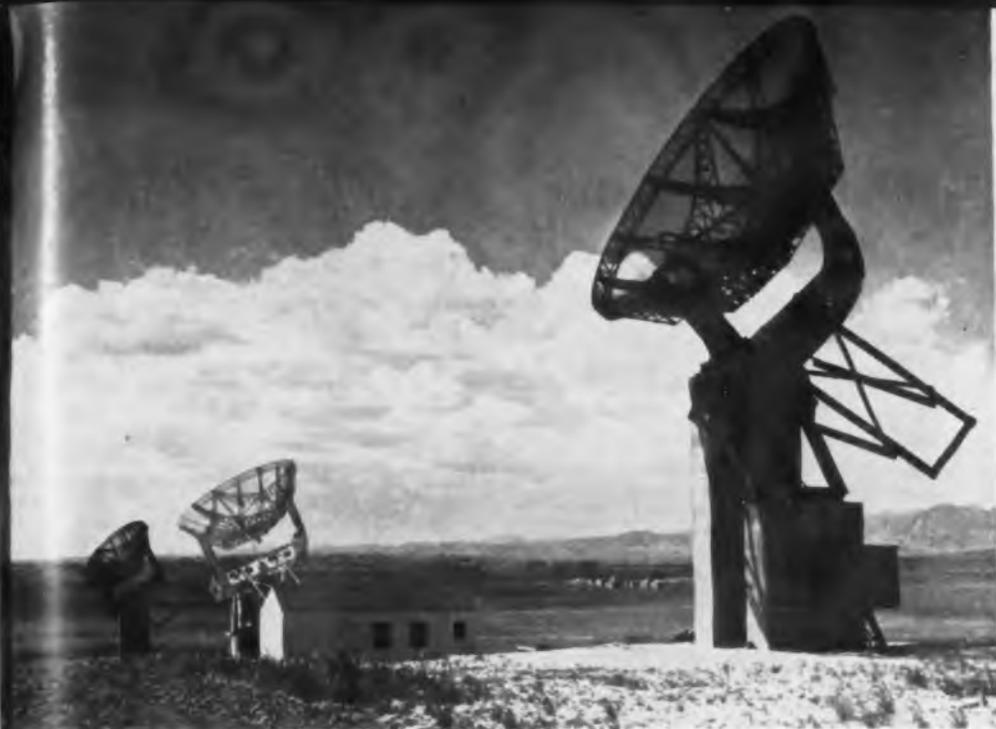
Three giant Wurtsburg antennas at Gun Barrel Hill, Colorado, NBS field station, are arranged to receive signals of a certain frequency radiated from the sun and to track the sun across the sky
