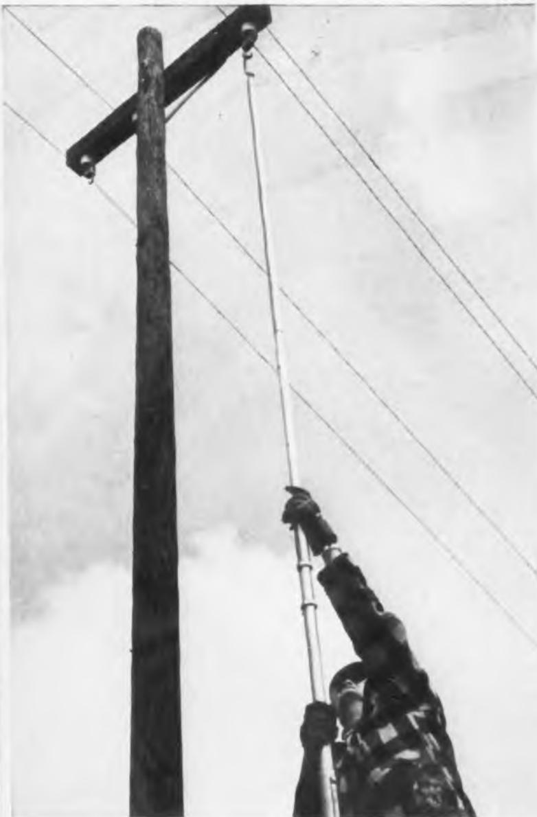
*Fastening wires with new tool.*
