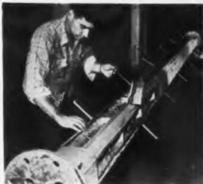
UMF-TV transmitting antenna windows at Gabriel Co. are weatherproofed with solid sealer made by Minnesota Mining & Mfg. Absence of solvent eliminates possibility of shrinkage
