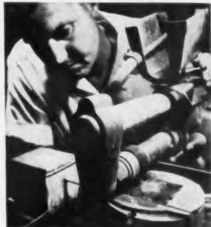
Rate grown transistor ingot is diced by means of ganged diamond saw at General Electric. Bars on glass plate will become transistors by simply attaching leads at ends and middle
