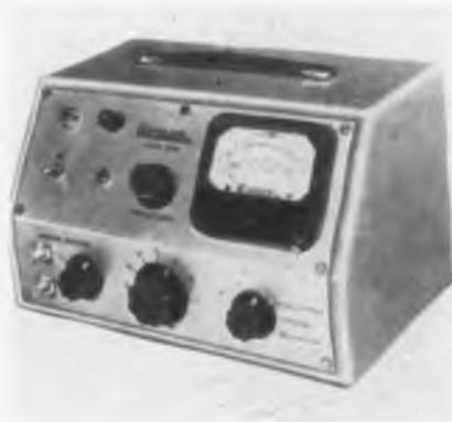
eliminate continuous cable changes. sensitivity 0.3 mv for full scale deflection, 60 db range calibrated to  $\pm 0.1$  db/10 db step, crystal or bolometer inputs, plug-in filter units from 250 to 2500 cps. The culmination of extensive research, it is said, the unit affords greater ease of operation with faster and more accurate readings. **Waveline, Inc., Greenbrook Rd., Caldwell, N.J.—TELE-TECH & ELECTRONIC INDUSTRIES.**
