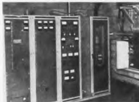
Three-cavity klystron transmitter on top of Cheyenne Mt., Colo. aids tropospheric research
