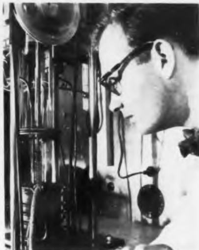
William Engeler, GE design engineer, checks first step in production of rate-grown transistors—crystal growing in furnace. Some 2000 units are made from single crystal ingot
