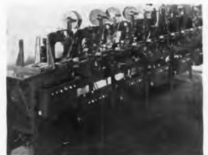
System for automatic assembly of electronic equipment employs several stations to insert various components in printed wiring boards
