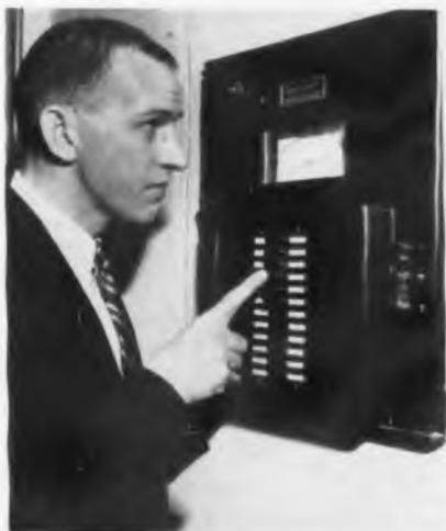
New cage-by-cage electronic heating control made by Minneapolis-Honeywell and installed in the reptile house of New York's Bronx Zoo lures the snakes to the front of the cage where they can best be viewed. Grading up of temperatures toward front encourages comfort-seeking creatures to move forward
