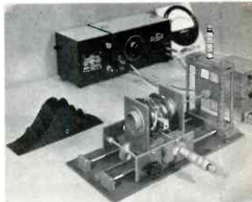
Equipment used to plot magnetic field inside deflection yokes. Note 3D field model!
