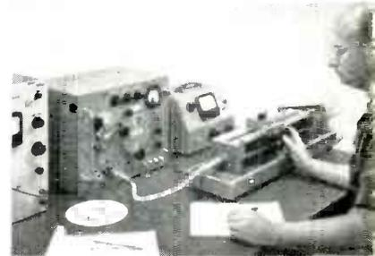
**Electronics Research Engineer F. R. Zboril** measures input impedance of a scale model helical antenna array used for ground tracking of missiles. Most of Lockheed's other antenna work involves advanced research studies on flush mounted antennas.
