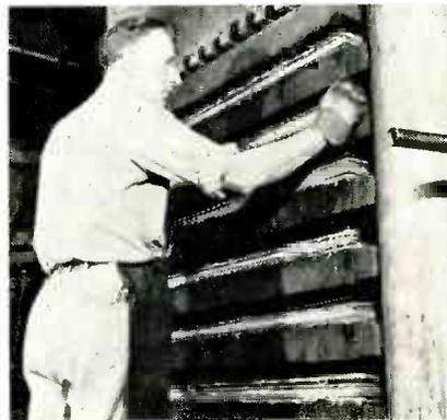
Fig. 3: Operator loads packs in 10 opening press. After one hour at 350° F and 1000 lb/sq. in. foil and laminate are bonded
