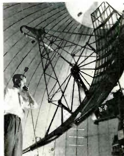
Inside radome building, radar height-finder has own room above control center. Air pressure supports rubberized glass fabric "balloon." Radome entrance is through air lock chamber
