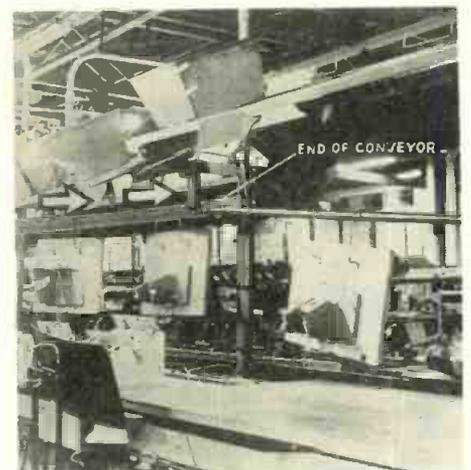
Rotating cable conveyor delivering empty pallets to slide rail storage
