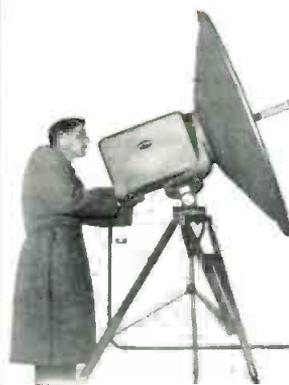
The ultimate in simplicity and portability, Raytheon KTR equipment for portable use consists of only four compact units with a total weight of 162 lbs. Portable units are available for all bands—color or monochrome with audio channel—if desired.
