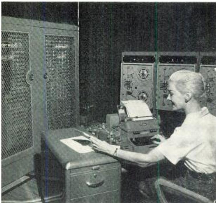
Newest in the line of electronic office equipment is this Underwood "ELECOM" File processor which reduces the contents of 1600 conventional file cabinet drawers to less than 3 cu. ft. of space. The unit also feeds desired information via tape to a companion computer.
