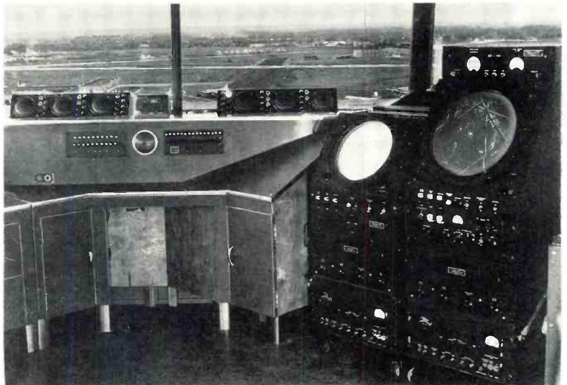
Fig. 2: (r) Experimental model of ASDE installed in the control tower at Idlewild
