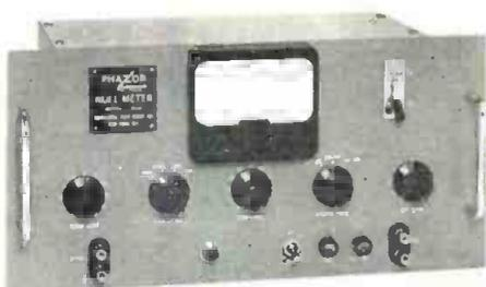
ance; and electronic limiting to prevent instrument overload. Power input is 105-125 v, 60 cps, 25 w. Industrial Test Equipment Co., 55 E. 11 St., N.Y.C. Tele-Tech & ELECTRONIC INDUSTRIES (Ask for 6-114)
