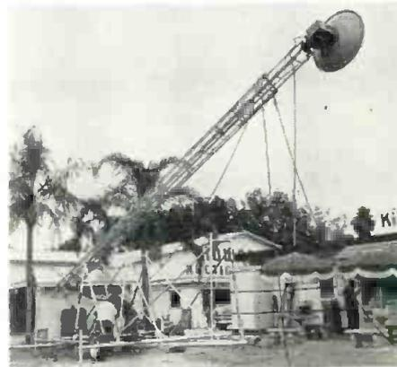
leaving the ground. WFLA-TV has been using this new tower on a remote pick-up 20 miles from its station, with outstanding results. **E-Z Way Towers, Inc., P.O. Box 5491, Tampa, Fla. TELE-TECH & ELECTRONIC INDUSTRIES (Ask for 4-30)**
