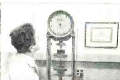
Quantitative checking of weld strength.
