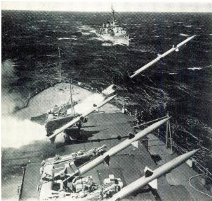
Navy's "Terrier" guided missiles are shown being launched from the deck of the U.S.S. Mississippi. Built by Convair Div. of General Dynamic Corp., for the Navy's BuOrd, Terrier is the Service's prime surface-to-air missile, designed to intercept aircraft at longer range and higher altitudes than conventional aircraft guns
