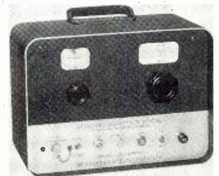
network of the Model 202-C contains a Bolometer which produces a resistance unbalance proportional to the signal. Measurements Corp., Boonton, N. J. ELECTRONIC INDUSTRIES & Tele-Tech (Ref. No. 10-18).
