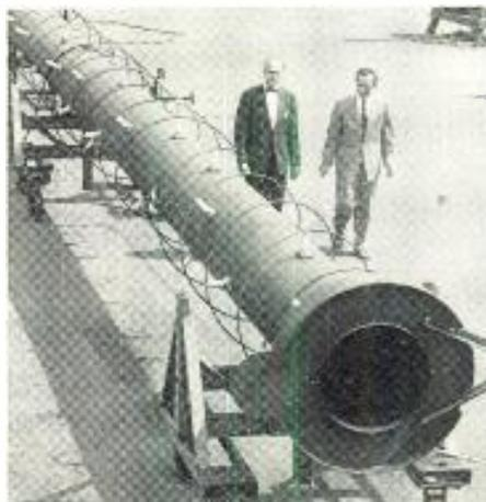
New high-powered VHF helical TV broadcast antenna developed by General Electric. Three-bay antenna features simplified design; it weighs 7,700 lbs., measures 80 ft. in length.
