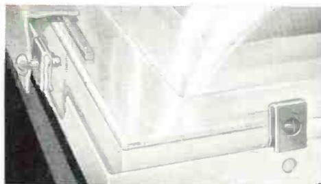
Assembly costs on this sheet-metal skylight frame are reduced 66% by Tinnerman "U" type SPEED NUTS.
