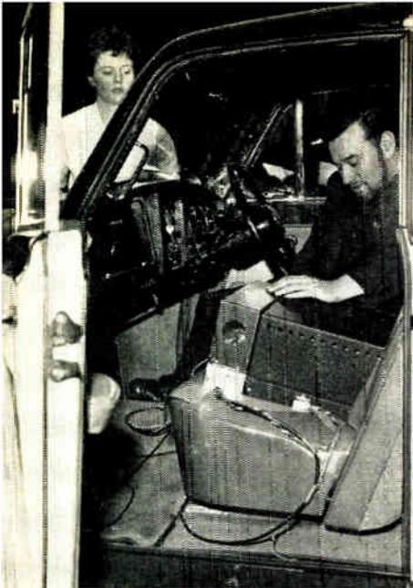
This telemetry transmitter easily fits into car which is undergoing testing. Up to 23 readings can be made simultaneously.
