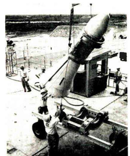
Re-entry vehicle traveled 1/3 of the way around the earth after being launched aboard an Atlas ICBM from Cape Canaveral. The Mark 3 was developed by GE's Missile and Space Vehicle Dept., Phila., Pa. Ablation materials absorb re-entry heat.
