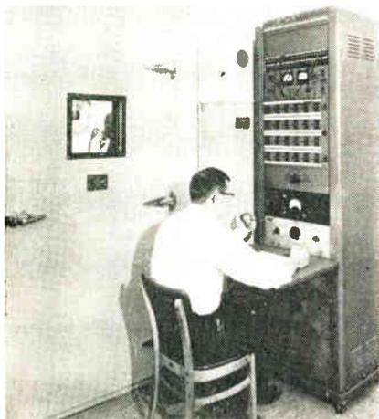
Insulated noise room, built by Shure Brothers, Inc., to aid development of better noise-discriminating microphones duplicates loudest sounds man can produce. Though generated sound inside is intense, D. O. Rail's voice is transmitted clearly, with background noise muffled. A. J. Brouns sits at the control panel, monitoring.
