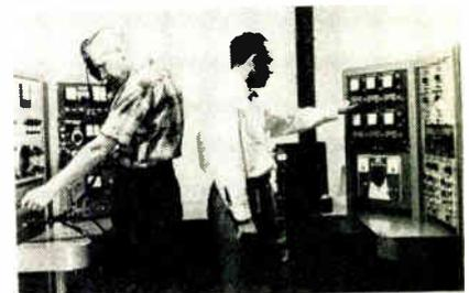
Instruments that record the pilot's bodily responses are checked by Armour Research Foundation technician, R. Fors and research scientist, E. S. Gordon. Designed by ARF for the Aero-Space Medical Div., Wright-Patterson Field, Ohio, they are used with a vertical accelerater.
