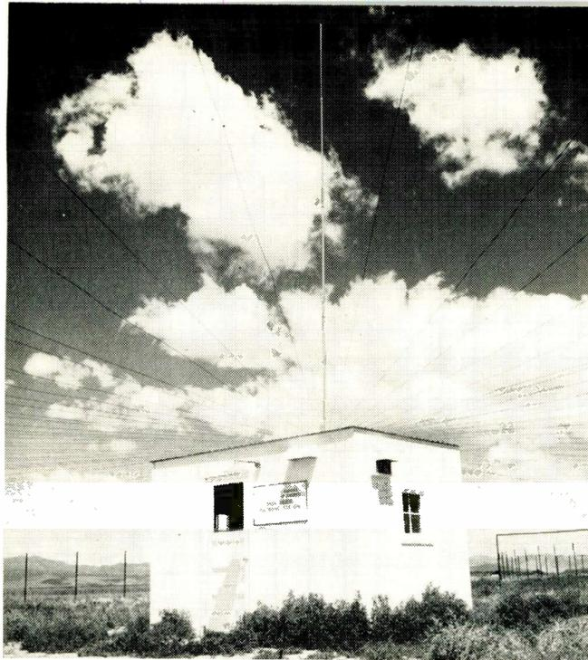
Fig. 1: Noise recording station typical of those set up by NBS during the International Geophysical Year. Data obtained from a world-wide network of these stations formed the basis for a graphical method which can be used to predict the characteristics of radio noise.
