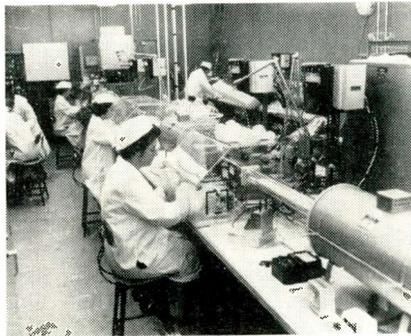
Transistors are now being manufactured in this new "controlled conditions" plant of National Semiconductor Corp., Danbury, Conn. The transistors in production are p-n-p silicon alloy "small signal" types for low power level amplification. Other types are planned for future production.
