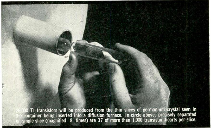
26,000 TI transistors will be produced from the thin slices of germanium crystal seen in the container being inserted into a diffusion furnace. In circle above, precisely separated on single slice (magnified 8 times) are 37 of more than 1,000 transistor hearts per slice.
