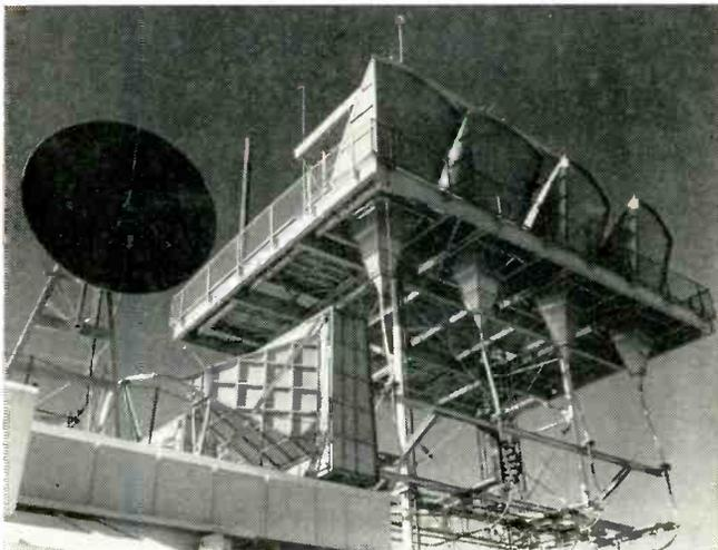
New high speed method of transmitting scientific and business data by microwave is now being used by North American Aviation, Inc. Dish at left on Oat Mountain receives microwave signals from Rocketdyne, 9 miles away, then beams them to Los Angeles 30 miles away.
