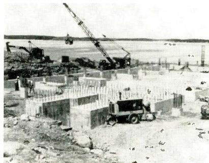
Power plant foundations. Five large blocks run at right angles to the length of the building. The two small blocks (left, foreground) are foundations for small generators.
