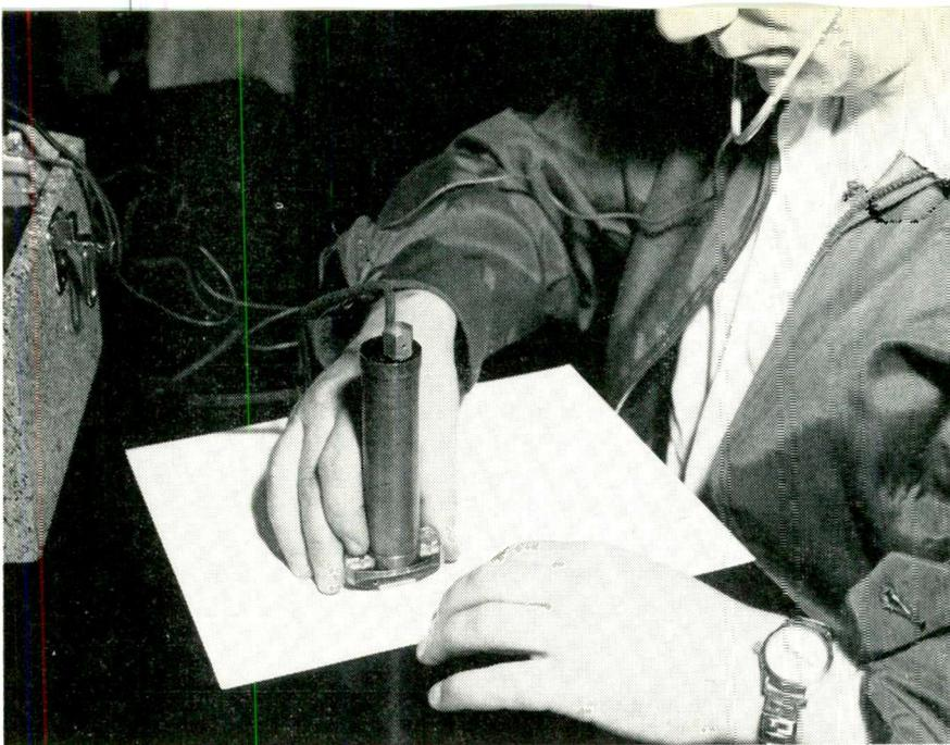
Fig. 9: This Aural Reading Device for the Blind, designed by Battelle's Engineering Psychologists will give blind people access to ordinary printed material. The device has 11 frequency channels and is "read" somewhat like reading code.
