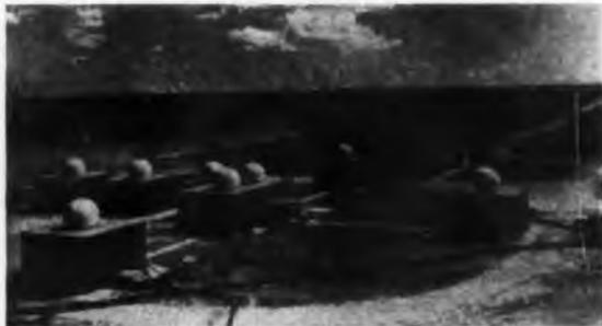
Battery of precision antennas inside cluster of white radomes at Cape Canaveral, Fla., enables Air Force to track missiles with an accuracy of a few feet at hundreds of miles. System is the Azusa Mark II, developed by Convair Div. of General Dynamics Corp.
