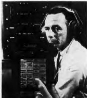
Communications device built by Hughes Aircraft Co. lets jet pilot "talk" to his base by punching indicated panels. Engineer Robert I. Harris demonstrates panel. Communications are twice as fast as normal and can penetrate heavy electrical interference.
