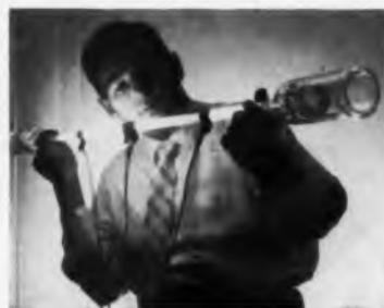
D. Herriett demonstrates technique for impressing telephone conversation on coherent beam of light generated by optical maser. Information handling capacity is millions of times greater than radio waves.
