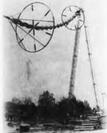
Seventy-four foot antenna insulator for the Navy's new radio station at Cutler, Maine, is tested on dummy tower at Lapp Insulator Co.'s High Voltage Laboratory in LeRoy, N. Y. System will be used with Polaris FMB system.
