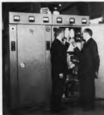
Continental Electronics Sales Manager T. Moseley, left, explains one of the new features of a 10 kw radio transmitter to A. Horvath, Radio Engineer for the Ecuadorian Government, which has purchased two transmitters from the Ling-Temco subsidiary. One transmitter will operate in the standard broadcast band, the other on shortwave.
