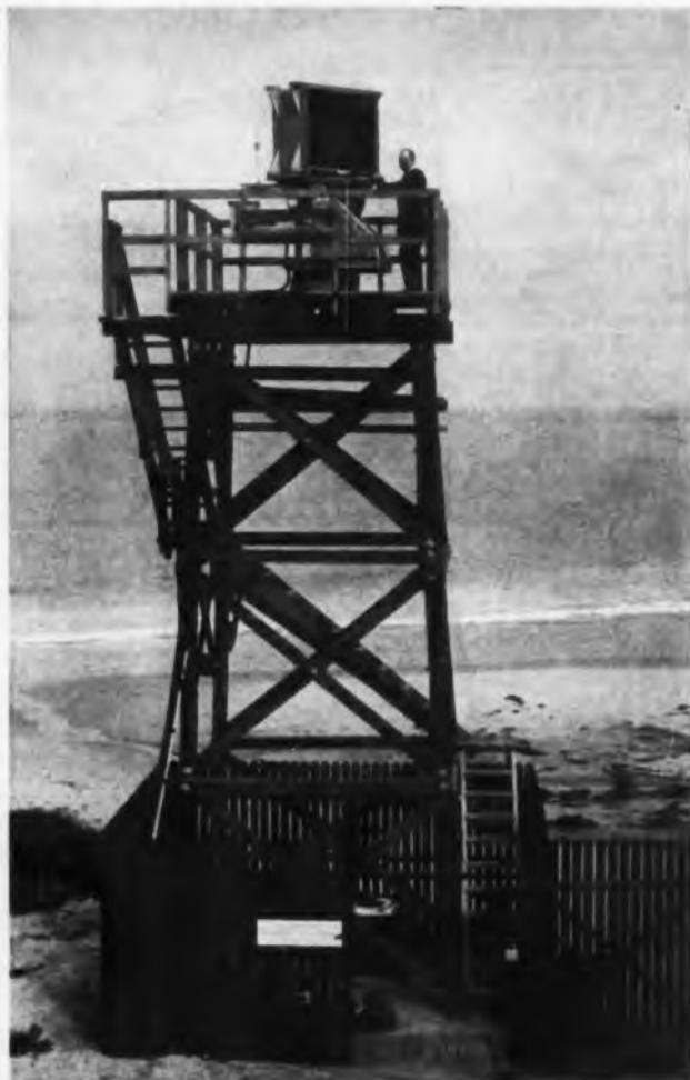
Before the new positioner was installed, the school was limited both as to size of antennas that could be tested and the flexibility of operation. Now, even in the face of strong winds, students can test big dishes and relatively large arrays of antennas: this particular model accepts a vertical load of 10,000 lbs. and has a bending moment capacity of 10,000 ft.-lbs. And with three axes, flexibility is virtually unlimited in taking "cuts".
