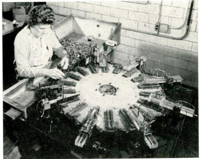
On this special automated equipment, a semi-skilled operator tests more than 2,000 custom-made, packaged assembly circuits per hour.
