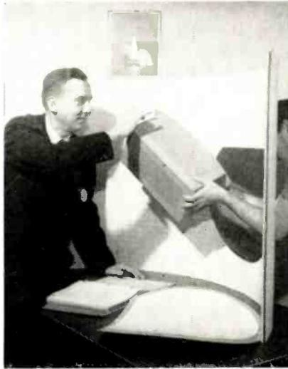
"How far is an arm's length?" Dr. Joseph W. Wissel is getting the answer with help of a mock-up of a section of a Polaris submarine launching tube. As a "human engineer," Dr. Wissel and his assistants at Lockheed Missiles and Space Co., prime contractor for the Polaris missile system, try to make it impossible for Navy technicians maintaining the missiles to make a mistake.
