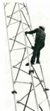
This tower is constructed in an equilateral triangular pattern of 3 1/2 ft. with the tower legs varying in tubular steel from 2 to 4 in. to meet the requirements of the installation. Tower is completely hot dipped galvanized and available for installations up to 800 ft. when using the proper size and weight of the tubular steel components. Can be tailored and engineered to meet exact needs of the antenna to be installed. Rohm Mfg. Co., Box 2000, Peoria, Ill.
