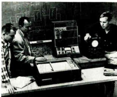
Robert D. LaRue, engineering professor at Colorado State U., shows use of general purpose analog computer and XY variplotter made by Electronics Associates, Inc. They are used in solving engineering problems. The devices will be used to illustrate the basic principles of flow and circuit diagramming, scaling and data presentation.
