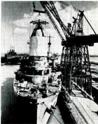
Three cranes load the prototype of Typhon Weapons Control System aboard test ship USS Norton Sound. Cloth-covered equipment, built at Westinghouse Baltimore Defense Ctr., is one of largest single pieces of electronic gear ever put on a Navy ship. The system will control anti-air missiles.
