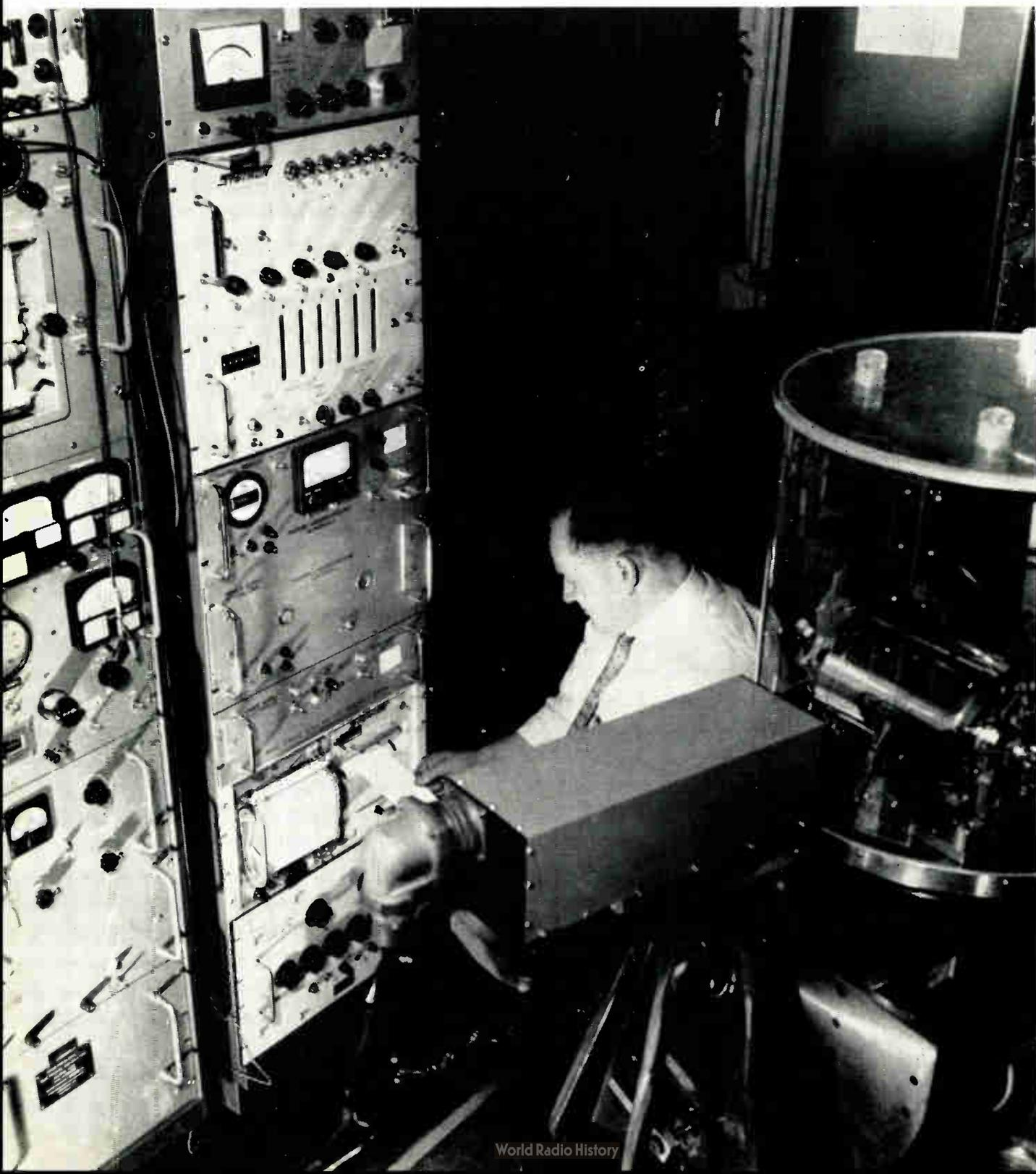
GYROS MUST BE TESTED AFTER THEY ARE BUILT TO learn how much they will drift. This drift must not exceed a specified rate or rejection occurs.
