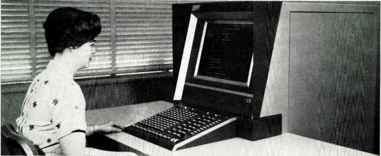
Message processing in the system described here includes queuing for display on electronic consoles such as the one shown above.
