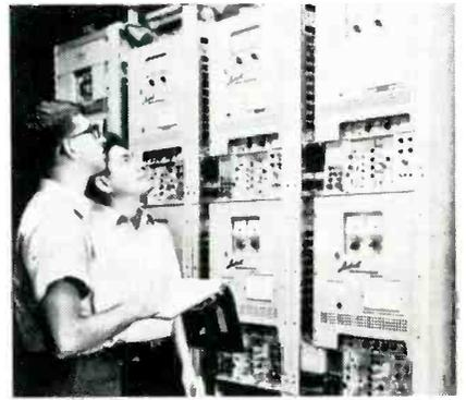
A 150-mile microwave radio system has been installed to consolidate communications for 53 U.S. and Philippine military commands and civil agencies, reports General Telephone and Electronics Corp. An AN/FRC-84 microwave terminal is inspected by a Navy technician (left) and a representative from Lenkurt Electronics Co., Inc., Division of GT&E, which installed the system on Luzon.
