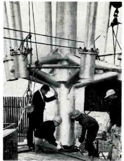
Non-destructive testing used on WBKB 174-ton TV mast atop Marina City tower in Chicago. Mobile test equipment from Magnaflux Materials Testing Lab use intense magnetic field set up in weld area dusted with ferro-magnetic particles to search out and detect any possible dangerous cracks in the metal. Erected by M&H Communications Co., the TV tower will reach 426 feet above Marina's roof and 1,000 feet above street.
