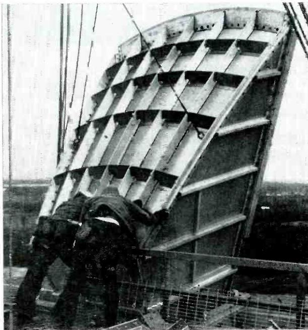
A.T.&T. engineers and workmen position section of large horn antenna on top of a TD-2 microwave radio relay tower near Mt. Royal, N. J., part of 54,000 miles of Bell's microwave network.
