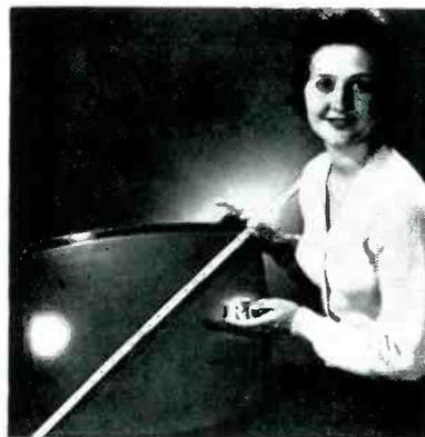
The aspect ratio on the screen has been adjusted to be more consistent with the standards of transmitter signals, giving a ratio of 3.12 to 4.0.
