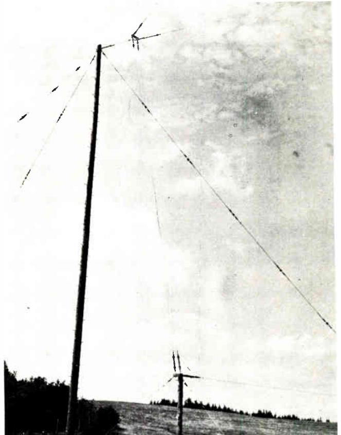
The input end of a common rhombic high frequency antenna.
