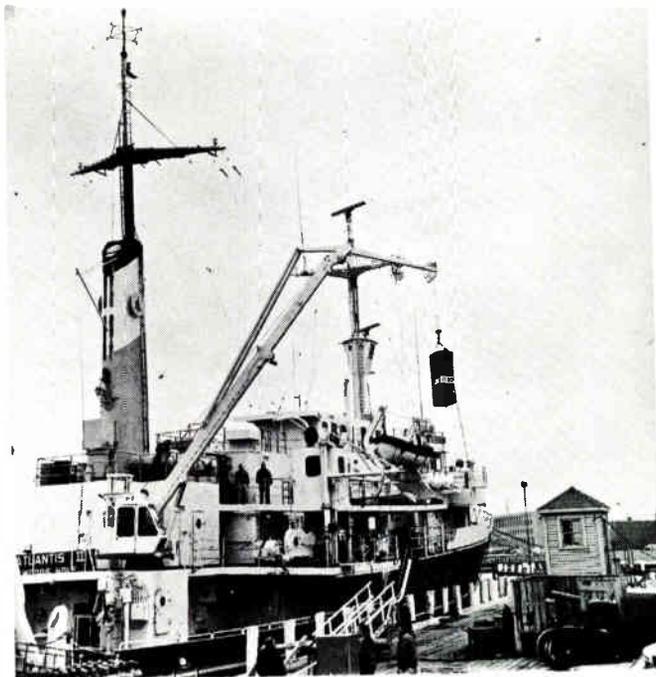
Part of a PDP-5 computer from Digital Equipment Corp. is swung aboard the Atlantis II, research ship of Woods Hole Oceanographic Institute. The computer will process ocean data and also will be used to navigate the ship by analyzing signals from satellites.
