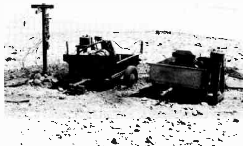
SO REMOTE is the Palm Springs translator site that all power must be "trucked in." The original generators were run on butane, while this pair operates from gasoline hauled to the top of the desolate peak.
