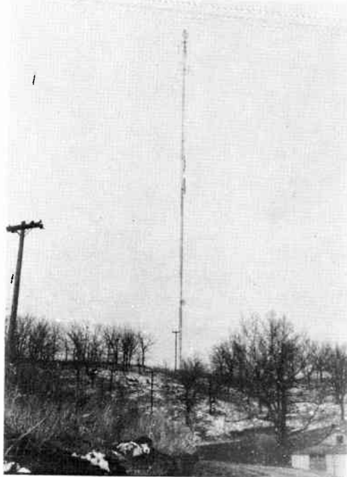
450 FEET ABOVE GROUND hidden in a swirling April snowstorm, the Redwood Falls, Minnesota receiving-transmitting tower looks anything but a "typical translator installation." Half way up—the transmitting antennas, at the top—the TACO ruggedized receiving yagis. Notes Klindworth, "I have over 400 TACO yagis in service, I've never had a major breakdown."
