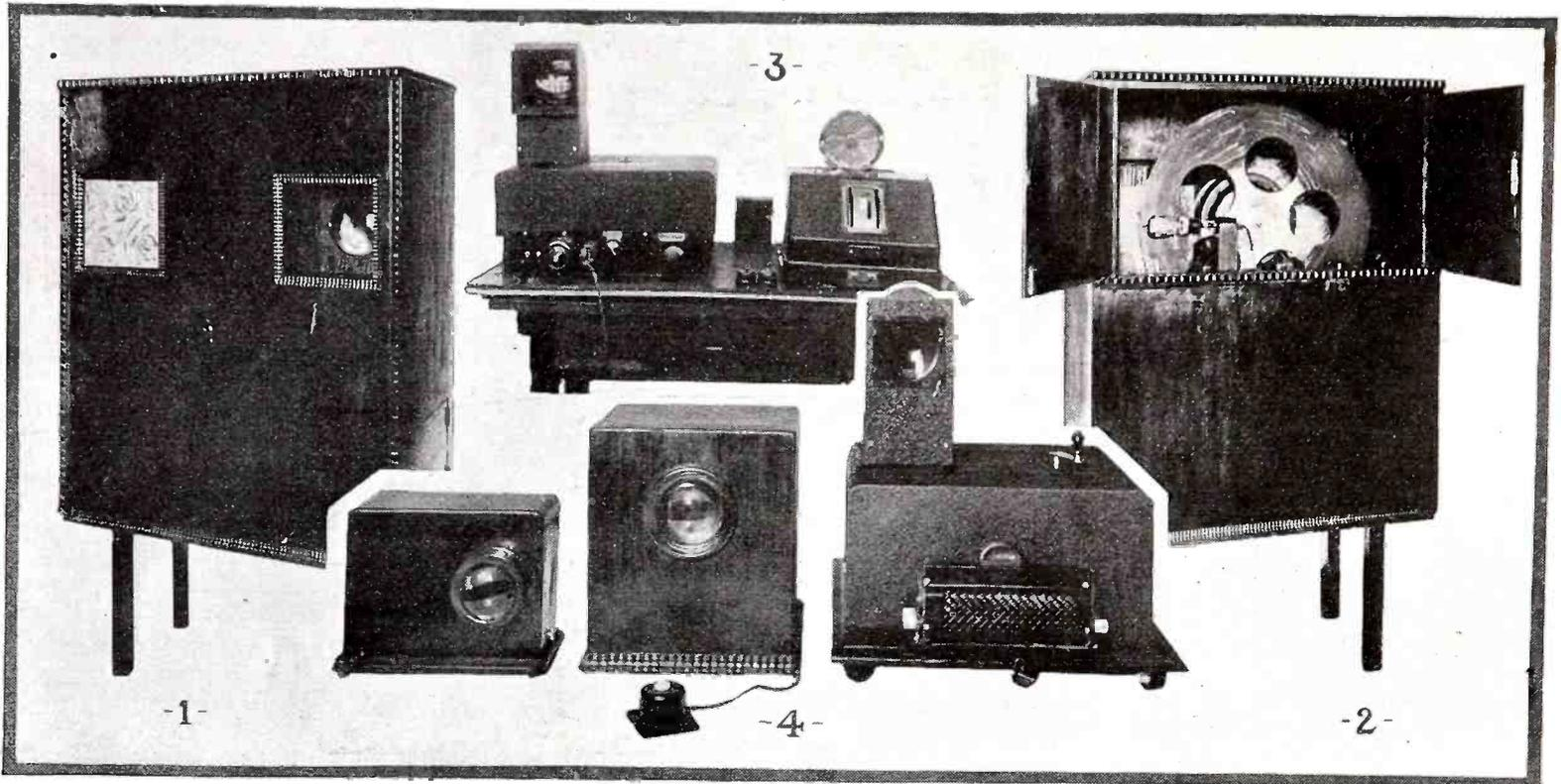
A group of televisions produced by the Telehor Company, of Berlin, which is developing the inventions of D. von Mihaly. The large sight-and-sound receiver shown at 1 is viewed from the rear at 2; it has a large disc, reproducing the image at the side in the window.
