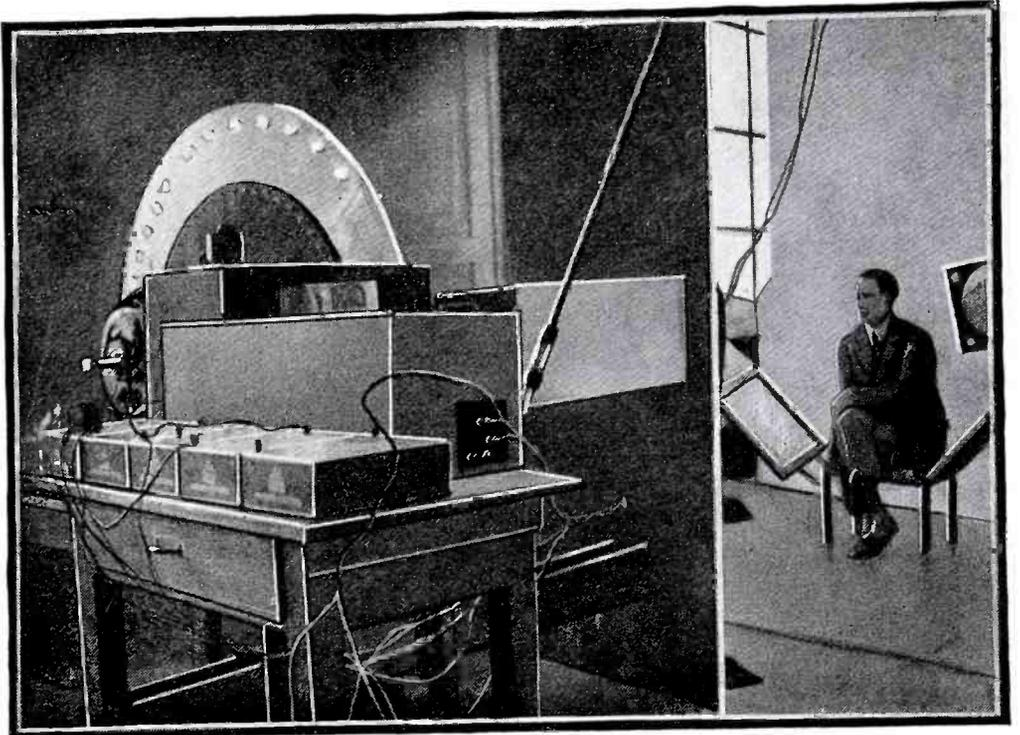
*The set-up of the Mihaly televisor for scanning subjects by natural daylight. Mirrors help to illuminate the subject properly; and a powerful lens concentrates the image upon the large scanning disc, which is placed in a dark room.*
