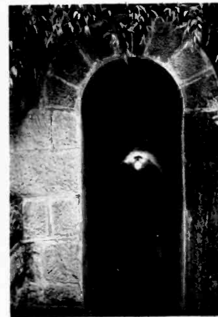
TUNNEL ENTRANCES to the underground caves which house the invaluable transmitters are concealed from air attack by camouflage.
