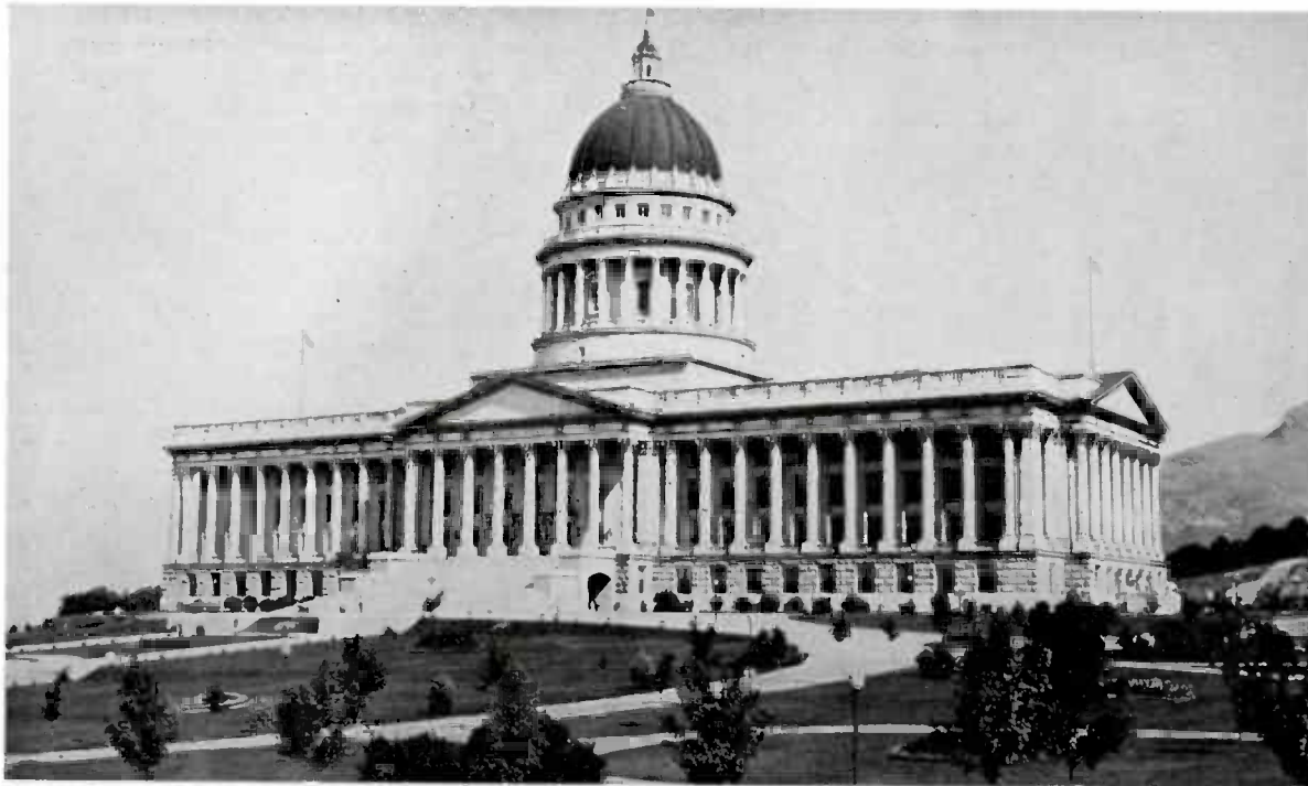
Utah State Capitol Building
