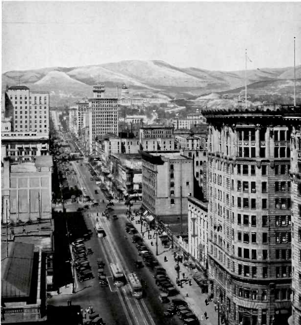
Looking North up Main Street
