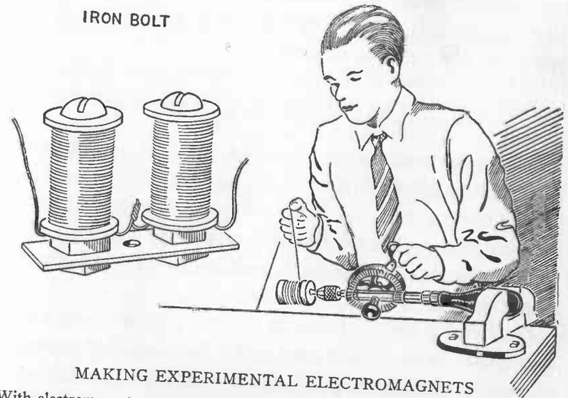
MAKING EXPERIMENTAL ELECTROMAGNETS
