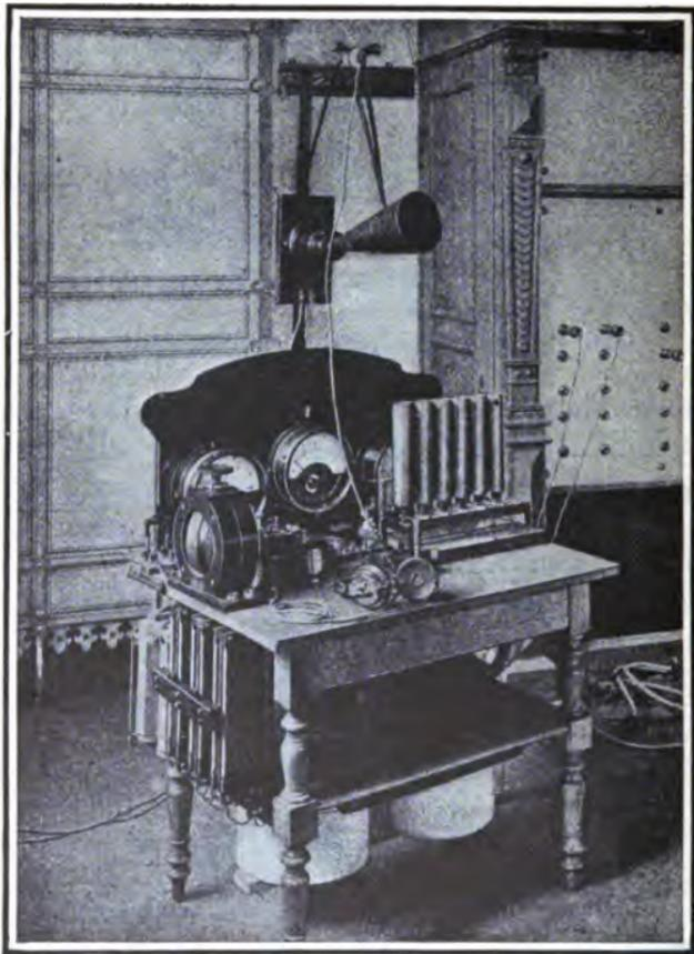
FIG. 147.—Poulsen wireless telephone equipment.
