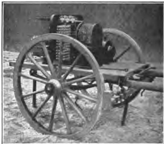
FIG. 101.—Telefunken wireless cart, showing transmitter.
