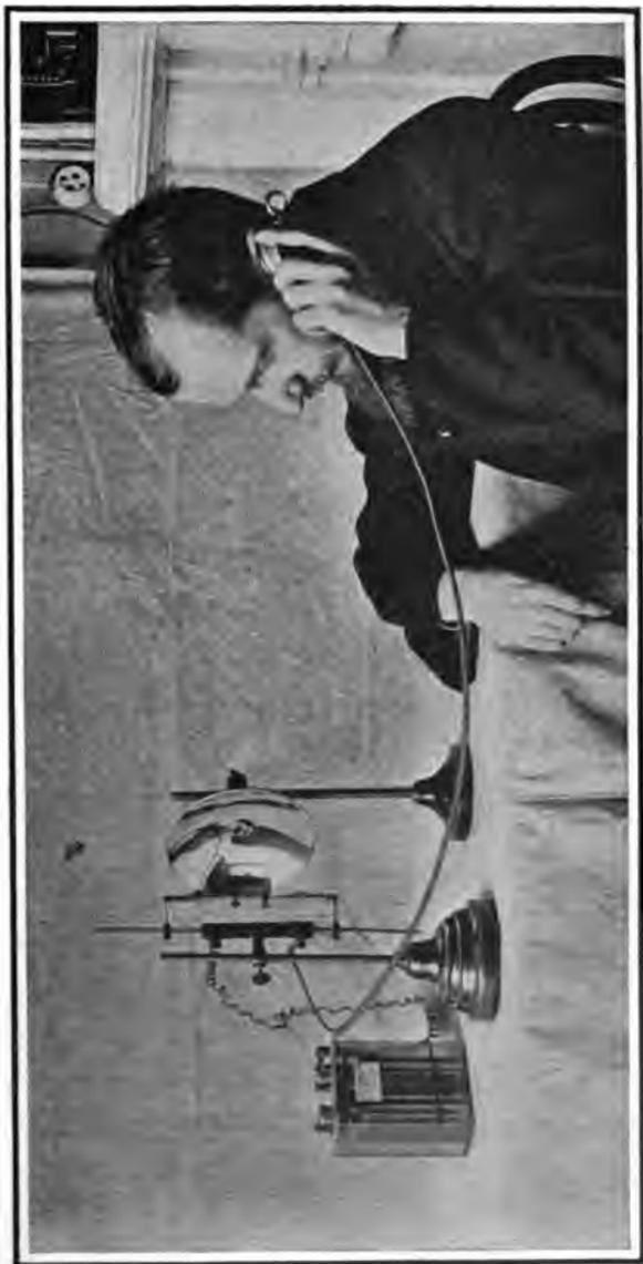
FIG. 134.—Photophone receiving apparatus.
