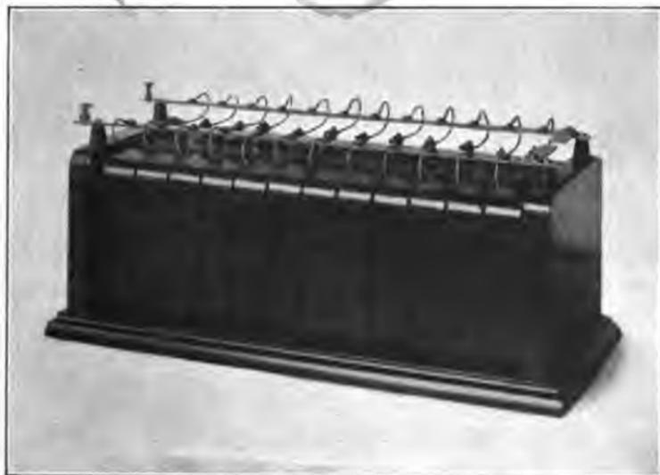
FIG. 95.—Transmitting condenser (molded dielectric).
