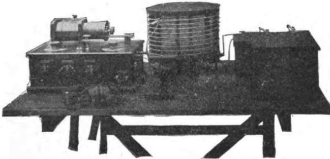
FIG. 99.—Complete receiving and transmitting outfit.
