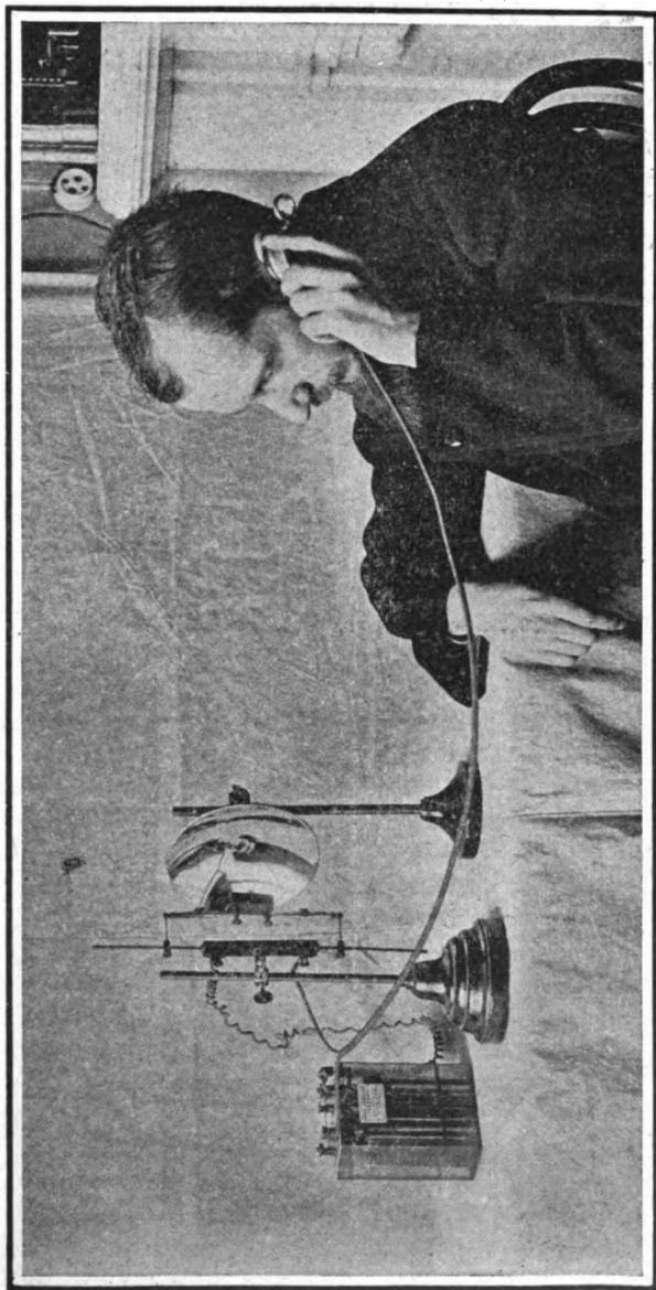
FIG. 134.—Photophone receiving apparatus.
