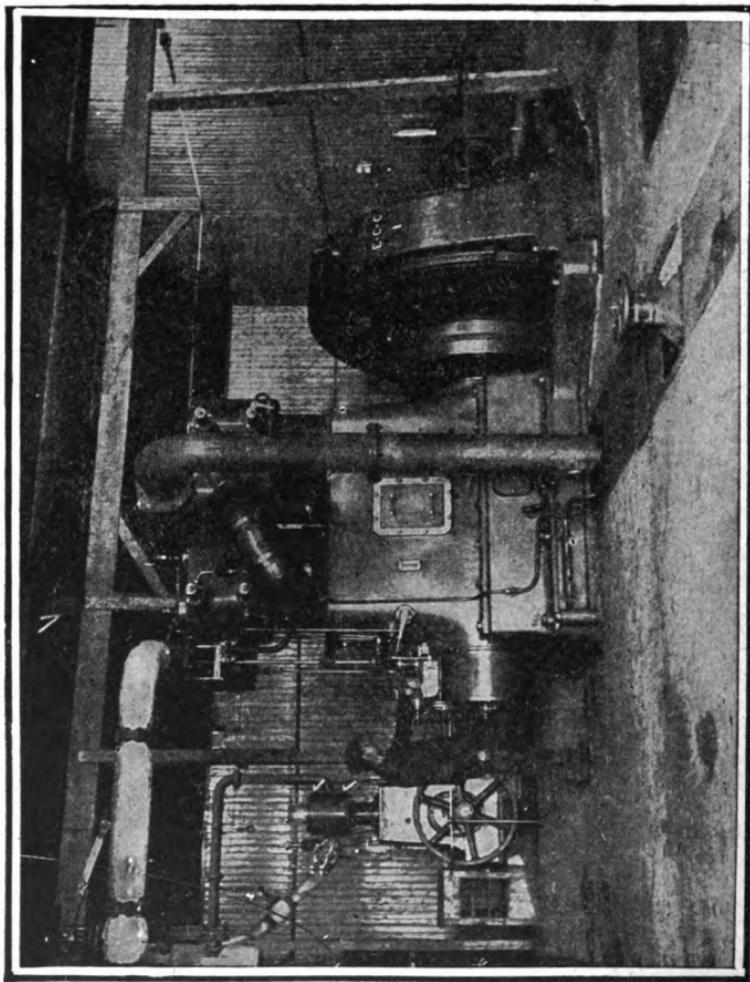
FIG. 29.—The power plant of a Marconi transatlantic station, showing engine and generator.
