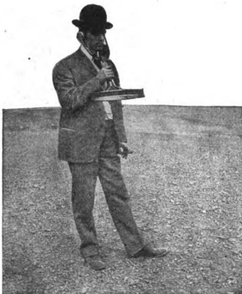
FIG. 141.—Wireless telephone receiving apparatus (induction method).
