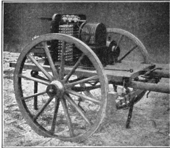
FIG. 101.—Telefunken wireless cart, showing transmitter.
