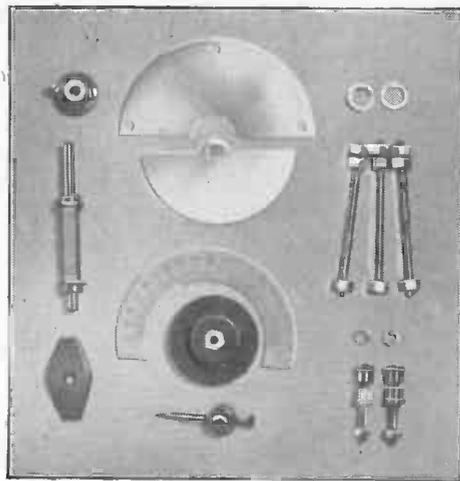
Fig. 162.—Parts of Variable Condenser
