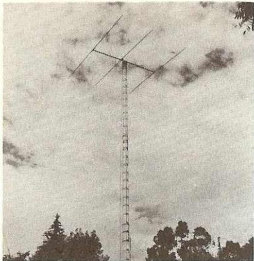
The use of rotary beam antenna is common practice in the amateur bands above 40 meters. A simple rotary array can quadruple the signal of the transmitter in the desired direction, and cut down on received QRM coming from unwanted directions. Shown at left is a three element 21 mc beam.
