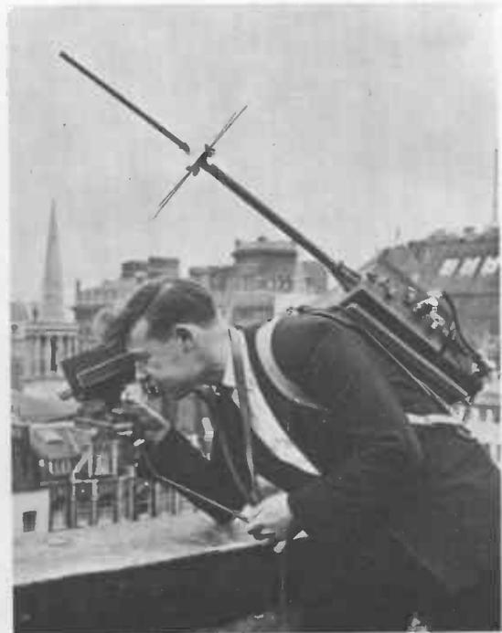
*Left:* Fig. 30 BBC Commentator Brian Johnston testing the portable Outside Broadcast amplifying equipment
