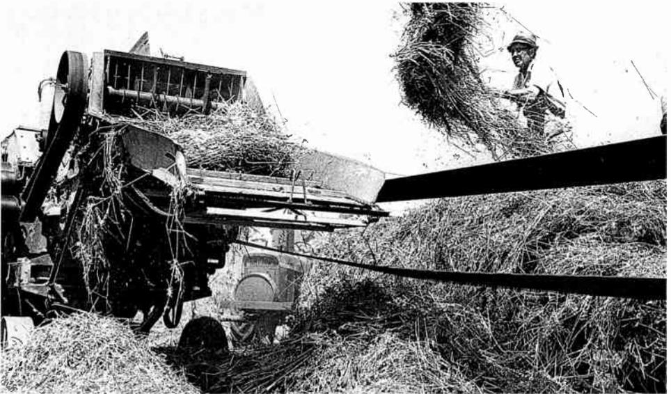
*Steam threshing in early 1970s. Robert Hale pitches grain bundle into the slat-belt feeder of the 36 inch Minneapolis grain separator. Machine is belt driven by steam engine 60-75 feet away, thus the long drive belt.*
