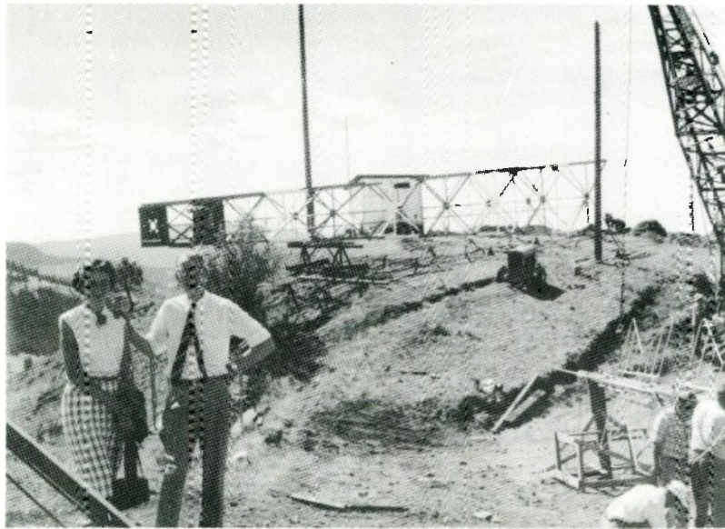
Sidewalk superintendents: The author and his daughter, Diane, watch a transmitting tower being erected on the peak of Mount Dufferin, west of Kamloops. It was a mystery to me that our engineering staff ever managed to get all the iron and steel material up the rugged mountain side, let alone erect it.
