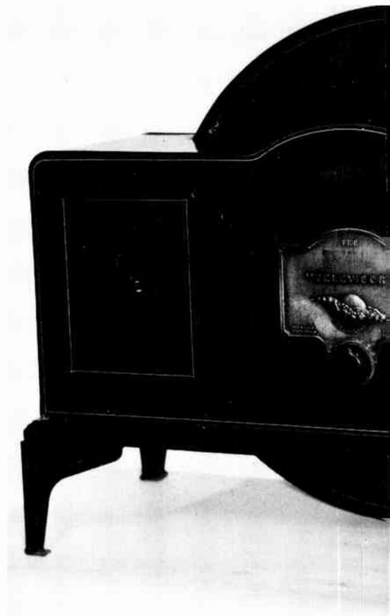
*Below A Baird Televisor. The picture was made of 30 lines, scanned vertically by Nipkow disc. The Plessey Company built 1,000 of these sets between 1929 and 1931.*
