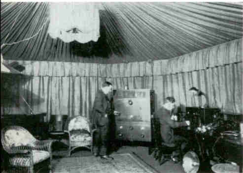
Station WDY established this broadcasting studio at Roselle Park, N.J., in 1921. One microphone was hidden in the chandelier; another in the cone suspended over the piano. The station amalgamated with WJZ, Newark, in 1922.
