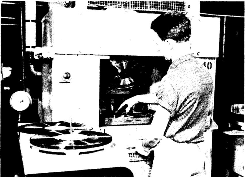
FIG. R/13. *Pressing the final record.*
