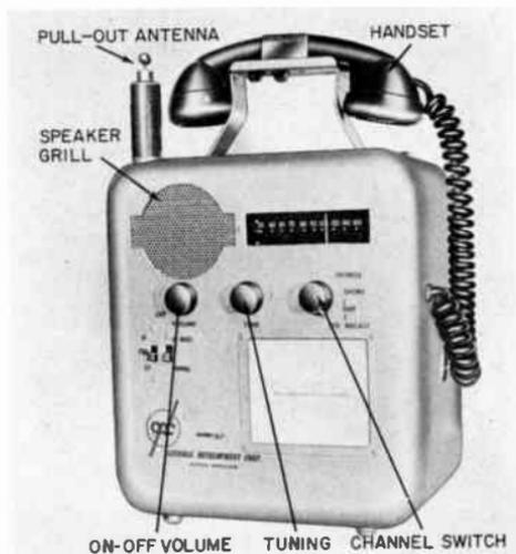
Fig. 306. A complete portable radiotelephone for shipboard use. It uses a telephone type handset and a collapsible antenna and will operate on distress frequency, shore or ship frequencies, and the standard broadcast band, depending upon the setting of the knob at the right. (General Development Corp.)
