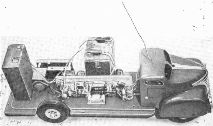
Fig. 1104—The receiver, batteries, and motor are mounted on the truck frame.
