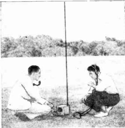
Photo at left—portable 5 and 10 meter combination "transmitter-receiver" in actual operation in the field. A telescopic antenna is very desirable for the purpose. Plate and filament supply is readily obtained from batteries.
