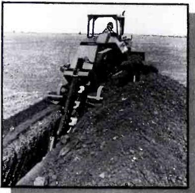
*Ditch Witch: conveyor spoils delivery system*
