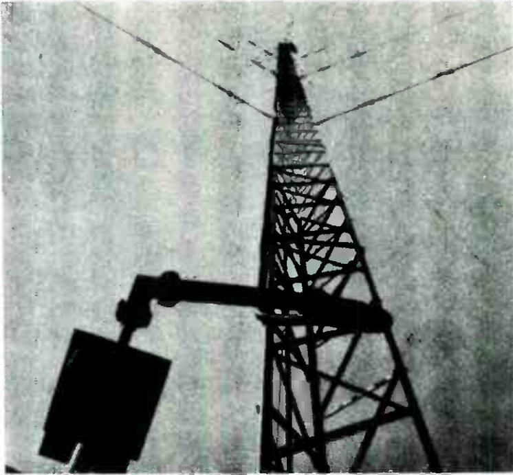
View of 326-ft Collins 37M-11 a-m tower with isolation coupler in foreground. The 11 bays of fm antenna are mounted at the extreme top of the tower.
