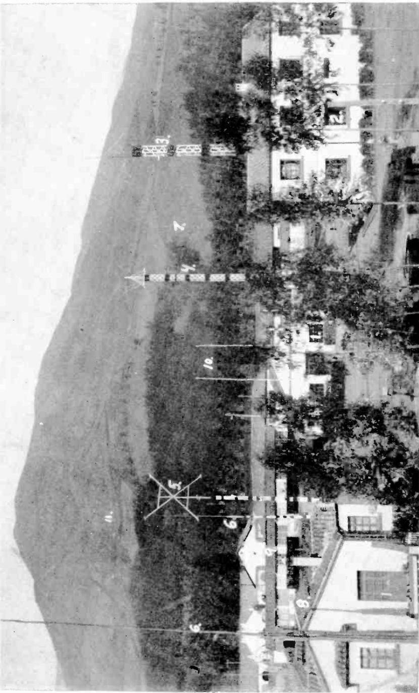
HCJB GROUNDS: 1. Transmitter Building, 2. Studio and Office Building, 3. 24-meter Tower, 4. 31-meter Tower, 5. 19-meter Tower, 6. Long-wave (308) Antenna, 7. 49-meter Antenna, 8. Co-directors' Home, 9. Bodega Apartments, 10. Flagpoles, 11. Mt. Pichincha.
