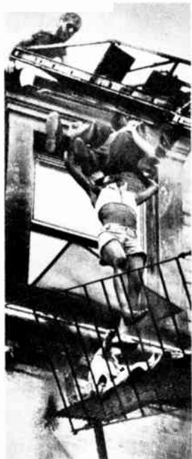
Fire Escape Collapses Under Victims
