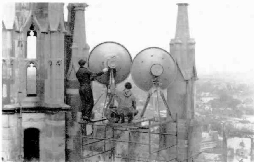
*Two micro-wave radio link engineers send back a signal from the top of Canterbury Cathedral to the Southern Television Centre at Southampton*
