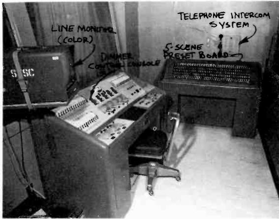
**8-10** Lighting Control: The lighting control board consists of the dimmers and their preset controls, through which a variety of lights can be adjusted for their intensity either individually or in unison, depending on how they are patched.
