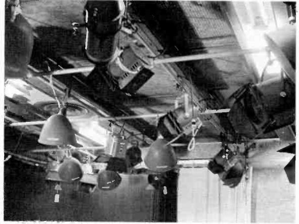
**5-31 Pipe Grid:** The pipe grid consists of rather heavy pipe strung either crosswise or parallel and mounted from 12 to 18 feet above the studio floor. The height of the grid is, of course, determined by the studio ceiling height, but even in rooms with low ceilings, the pipe should be mounted approximately two feet below the ceiling so that the lighting instruments or the hanging devices can be easily mounted onto the pipe.
