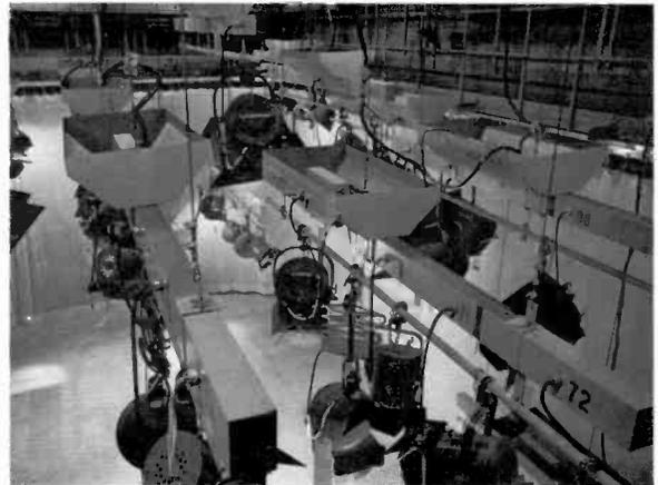
does not altogether eliminate the use of a ladder. Especially in small studios, the studio floor is rarely sufficiently clear of cameras, microphone booms, or scenery for the battens to be lowered all the way to comfortable working height. You will find that after having adjusted the lighting instruments as to direction and beam focus, you will still need a ladder or the lighting pole for the accurate final trimming once the battens have been raised to the proper position.
