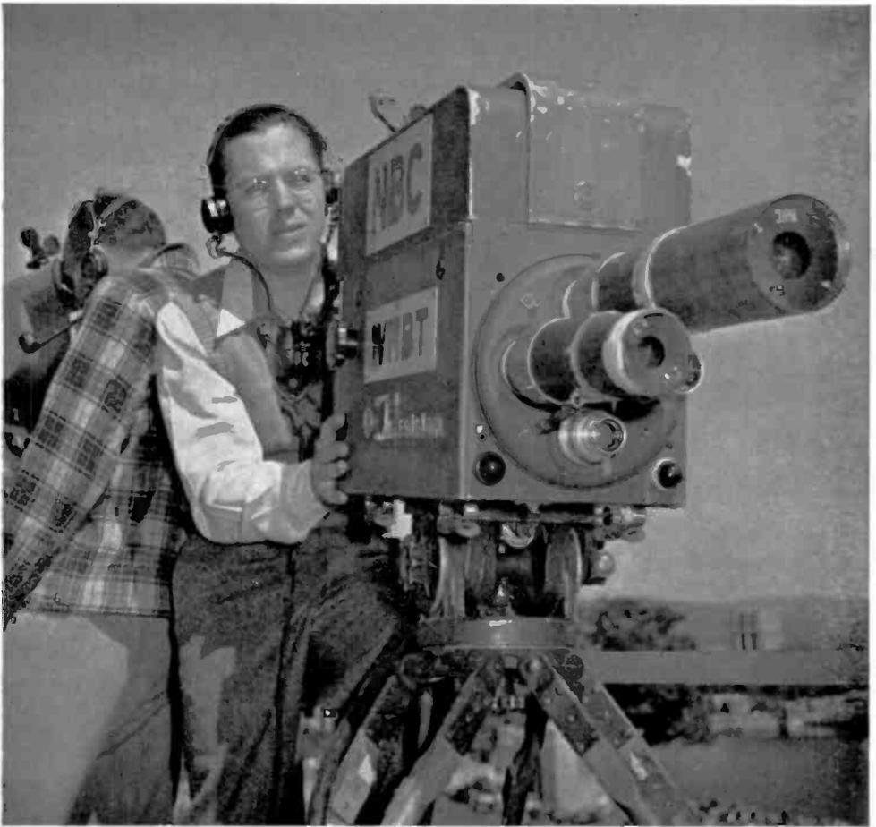
Typical television cameras in action during an outdoor telecast. The circular panel on which lenses are mounted is known as the turret. A simple mechanism throws the desired lens into action.
