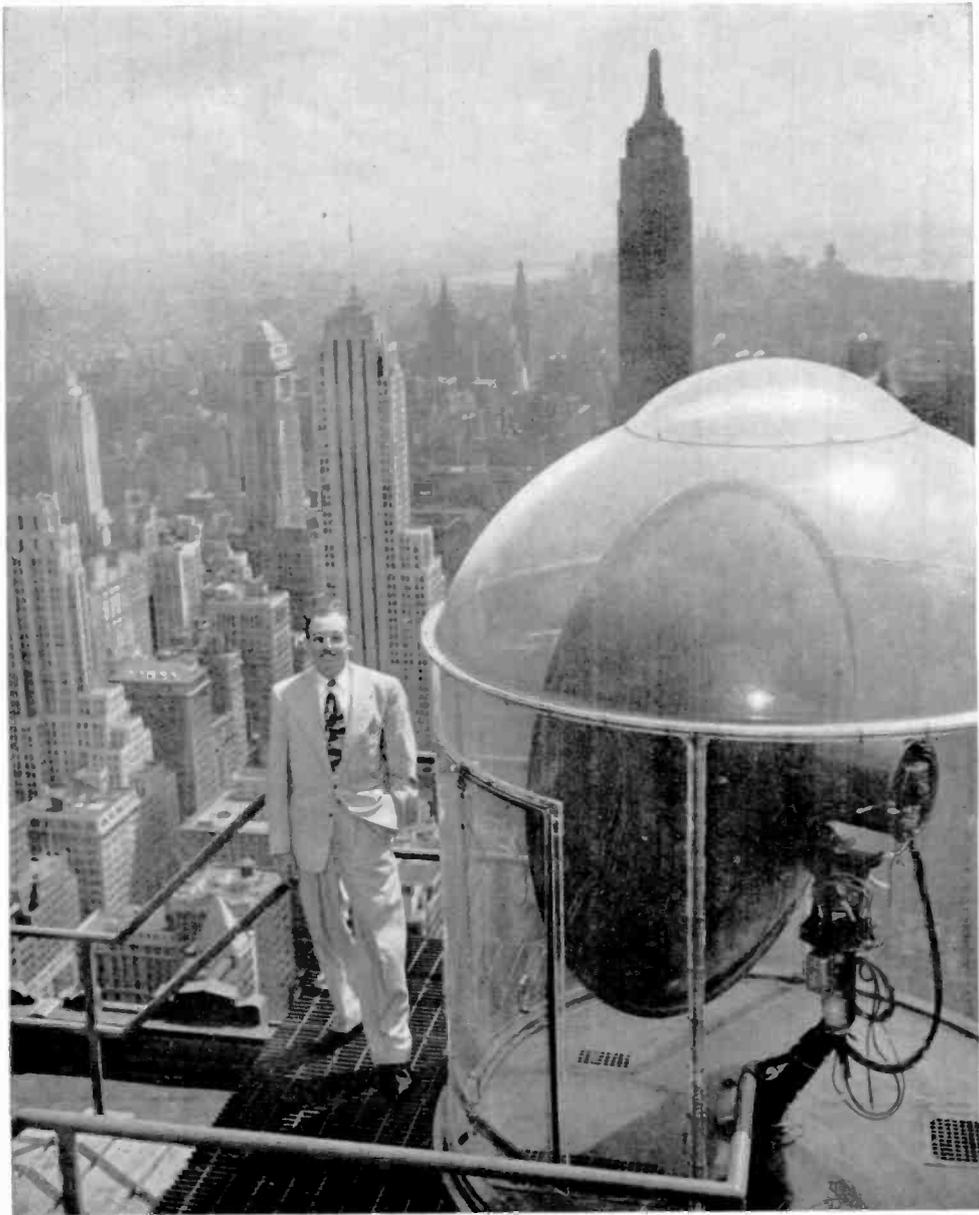
Chief Engineer O. B. Hanson, atop the RCA Building, inspects Radome, a parabolic antenna developed for microwave relay between New York and distant cities.
