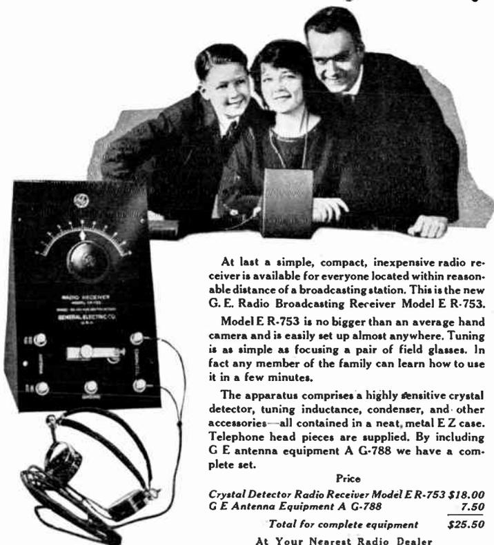
At last a simple, compact, inexpensive radio receiver is available for everyone located within reasonable distance of a broadcasting station. This is the new G. E. Radio Broadcasting Receiver Model E R-753.
